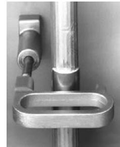
Rung protector installed showing proper placement.
