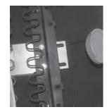
11. Route the conduit up to and through the access hole on the Rol-Loc's upper bracket to engage the pull release bracket attached to the top strap.
