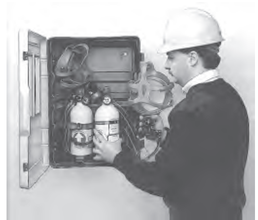
ESCBA units held in place with QUIC-RELEASE® straps.
