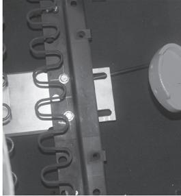
11. Route the conduit up to and through the access hole on the Rol-Loc's upper bracket to engage the pull release bracket attached to the top strap.
