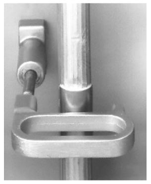
Rung protector installed showing proper placement. Old style handle assembly showing handle retainer casting.
